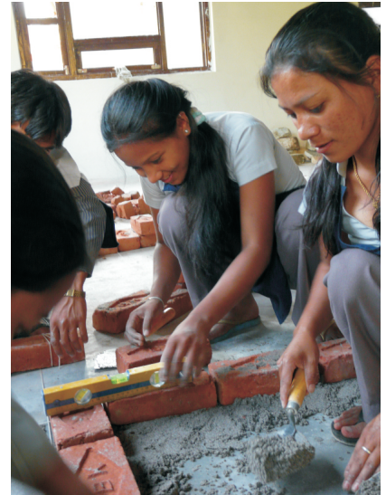
....and plastering a wall at the Gairi Campus.
